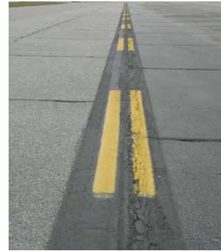
**Surface Painted Signs** are among other markings appearing on taxiways to augment vertical and lighted signs that are positioned along the taxiway edge. Surface painted signs aid the pilot and other drivers during low visibility conditions when the signs may be difficult to see, or when a taxiway exceeds certain widths; they can provide guidance information to an operator.
