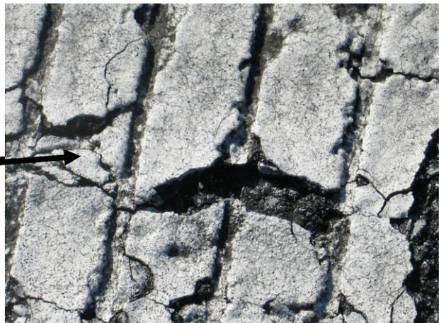
**FIGURE 5-5. MAGNIFICATION OF CRACKED MARKINGS AND ASPHALT FROM FIGURE 5-4.**
