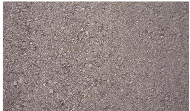
**FIGURE 4-10. AFTER RUBBER REMOVAL.**
