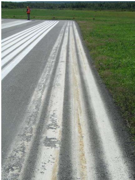
**FIGURE 6-16. LAYERED STRIATIONS ON THE SIDELINE WERE SCRAPED OFF BY SNOWPLOWS.**
