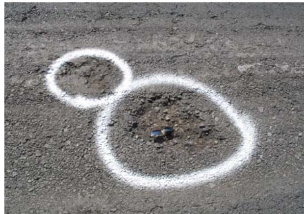
**FIGURE 5-24. PRE-EXISTING CONDITION CAUSED BY OIL SPILL ON ASPHALT.**
