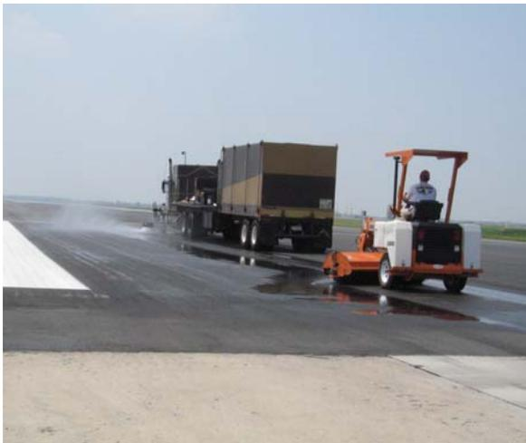
**FIGURE 5-31. CLEANING THE REMOVAL SCAR BEFORE APPLICATION OF NEW MARKINGS.**
