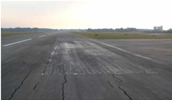
**FIGURE 4-16. BEFORE WATERBLASTING: ALGAE OBSCURE MARKING.**
