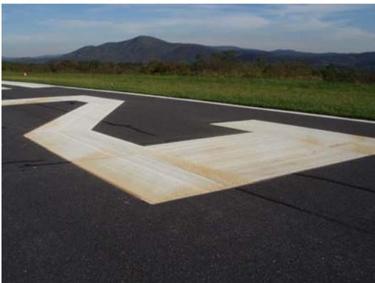
**FIGURE 4-29. REPAINTING WITHOUT CLEANING THE STAIN RESULTS IN BLEED-THROUGH.**
