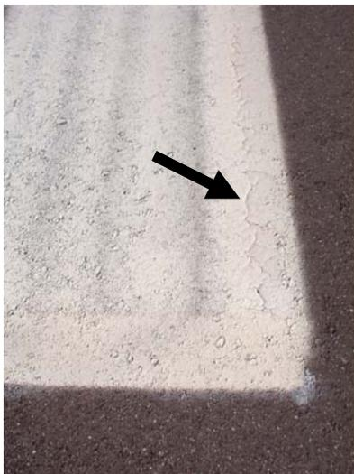
**FIGURE 4-11. PAINT CRACKS WHEN APPLIED TOO THICKLY.**
