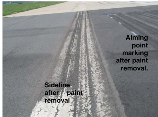
**FIGURE 5-27. BEFORE PAINT REMOVAL. FIGURE 5-28. AFTER PAINT REMOVAL.**
