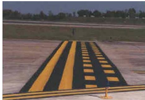
**Intermediate Holding Position Marking** is a “taxiway/taxiway” hold marking, designed to provide a place on a taxiway for a pilot to wait for another aircraft taxiing on an
