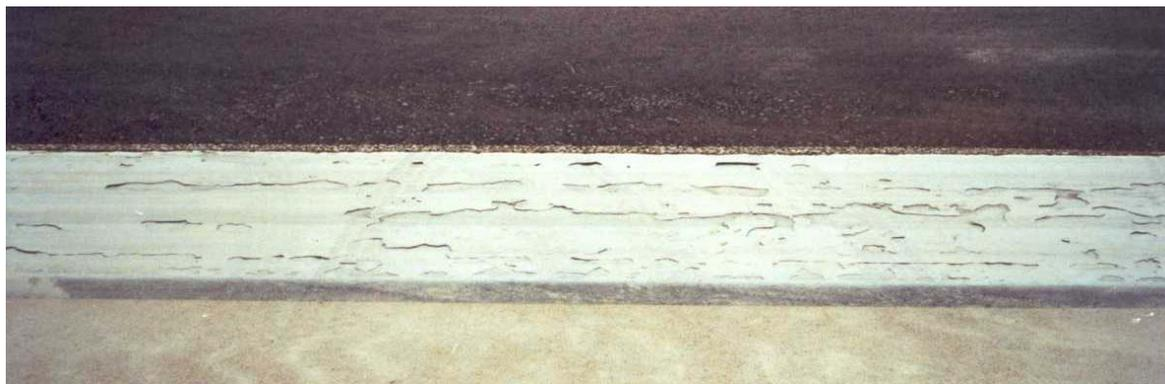
**FIGURE 4-3. REPEATED PAINTING ON CONCRETE LEADS TO FOD.**
