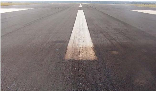
**FIGURE 4-32. THE OILY STAIN WILL PREVENT NEW COATING FROM BONDING.**
