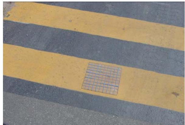
By using these three evaluations, one can determine whether or not the paint marking passes or fails. If the readings for any one of the three tests (the chromaticity, retro-reflectivity, or percentage of coverage) fail, **the pavement marking automatically fails.**
