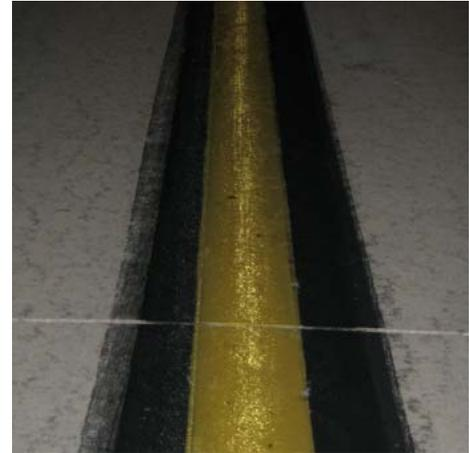
**FIGURE 3-9. NON-FUNCTIONAL MARKING DUE TO POOR REFLECTIVITY.**
