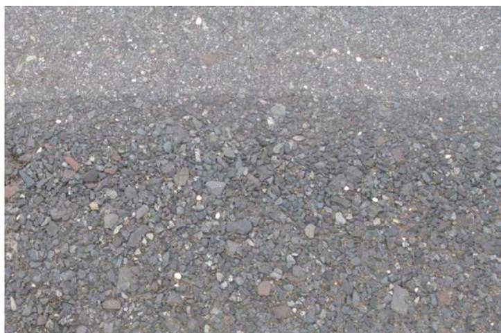
**FIGURE 5-25. REMOVAL OF MARKINGS FROM NEW ASPHALT RESULTS IN EXPOSED AGGREGATE (SCARRING).**
