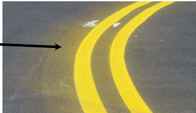
**FIGURE 6-45. CLOSE UP OF OVER SPRAY IN FIGURE 6-44.**
