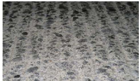
**FIGURE 5-17. AFTER TEN YEARS OF SHOTBLASTING TO REMOVE RUBBER DEPOSITS.**
