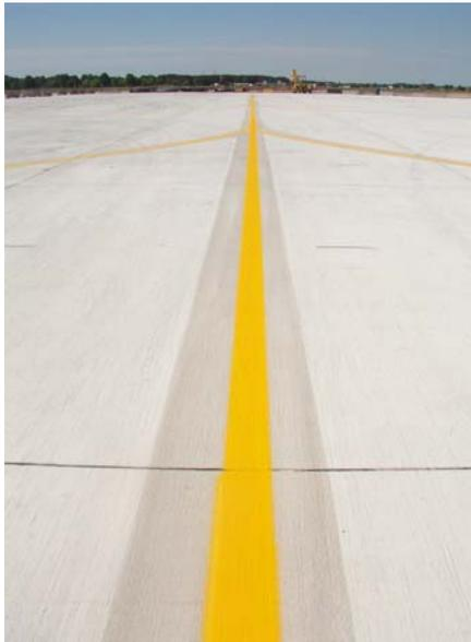
**FIGURE 6-1. CURING COMPOUND PROPERLY REMOVED FROM NEW CONCRETE.**
