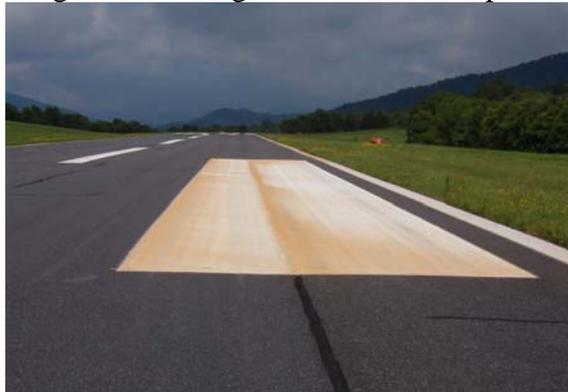
**FIGURE 4-24. STAINED LEADING EDGE AND LOW AREA ALONG JOINT WHERE WATER FLOWS.**
