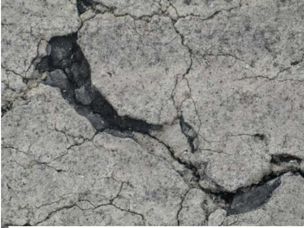
**FIGURE 5-29. CRACKED PAINT INDICATES PRE-EXISTING PAVEMENT DETERIORATION.**
