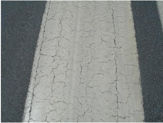
**FIGURE 4-6. THIS MARKING IS 30 MONTHS OLD AND CRACKED.**
