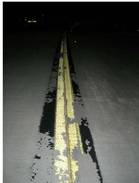
**FIGURE 4-8. EXAMPLE OF POOR REMOVAL OF CURING COMPOUND.**
