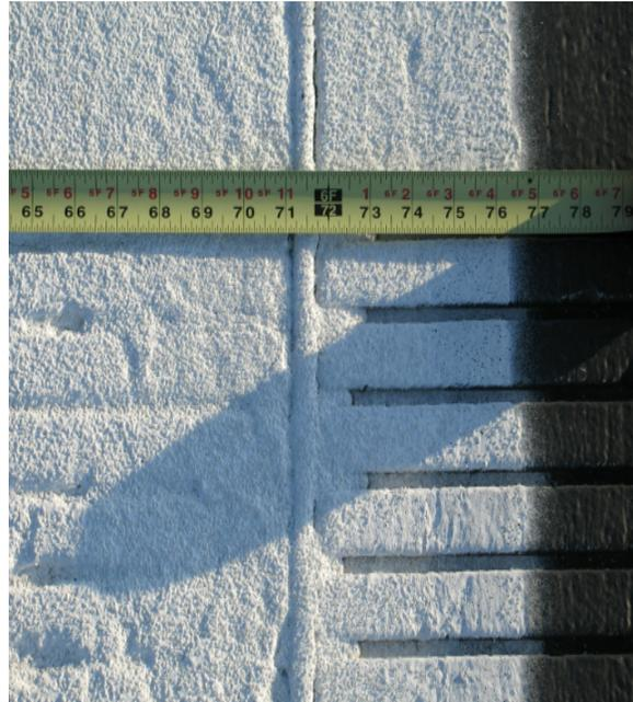
**FIGURE 2-3. MARKING DIMENSION IS OUT OF TOLERANCE.**
