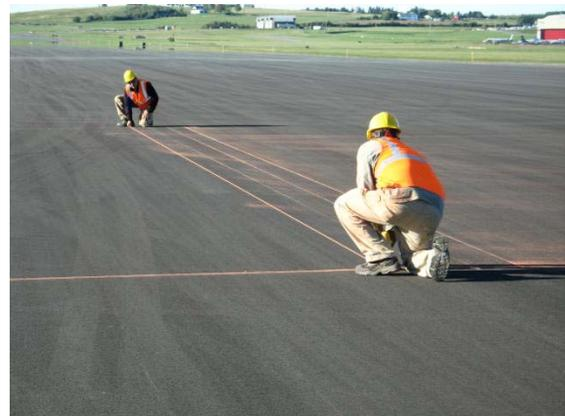
**FIGURE 6-3. LAYOUT WITH CHALK LINES ENSURES PROPER PLACEMENT AND ALIGNMENT.**
