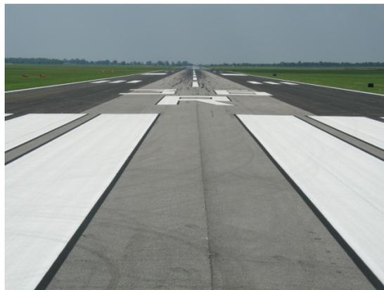
**Runway Centerline markings** designate the center of the runway. The centerline bars are measured from both ends toward the center; any irregularity in measurement is absorbed in the center of the runway, where it will be less noticeable.
