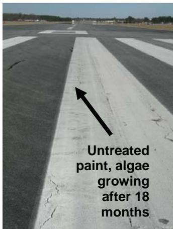
**FIGURE 4-18. PAINT USED WAS STANDARD TT-P-1952E.**
