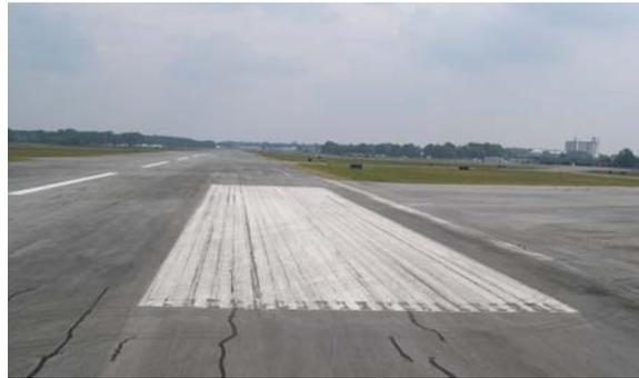
**FIGURE 4-17. AFTER WATERBLASTING, BUT BEFORE PAINTING.**
