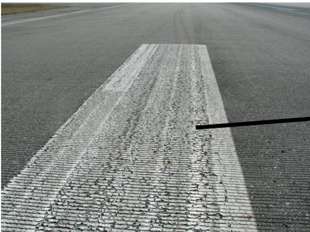
**FIGURE 5-4. CRACKED MARKINGS WITH DETERIORATED ASPHALT UNDERNEATH IS A PRE-EXISTING CONDITION.**
