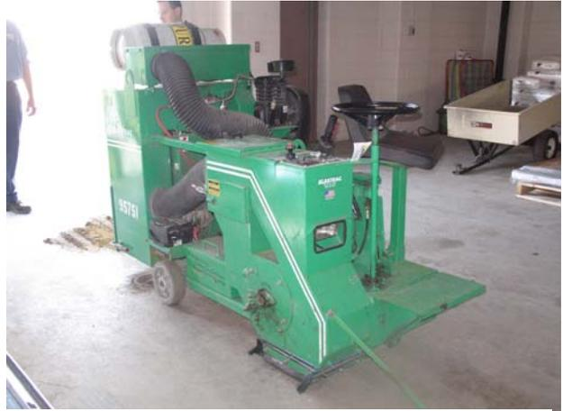
**FIGURE 5-13. SHOTBLASTER WITH A 10-INCH CUT.**
