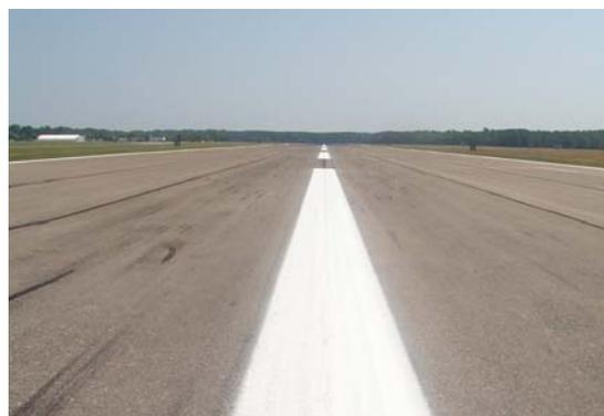
**Runway Threshold Bar:** Seen in the picture, “the threshold bar delineates the beginning of the runway that is available for landing when there is pavement aligned with the runway on the approach side of the threshold.” (FAA AC 150/5340-1J, page 6) All measurements for the aiming point and touchdown zone markings begin at the base of the **threshold markings**, not the threshold bar or edge of pavement.
