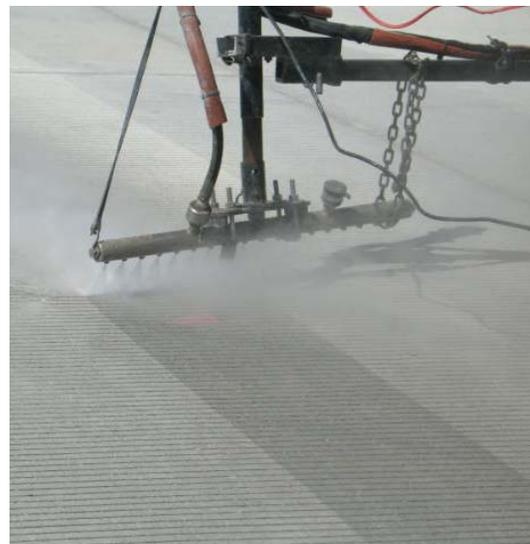
**FIGURE 4-38. LOW-PRESSURE WATERBLASTER.**
