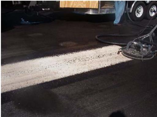
**FIGURE 4-34. THE PROCESS USED TO REMOVE OIL STAIN.**
