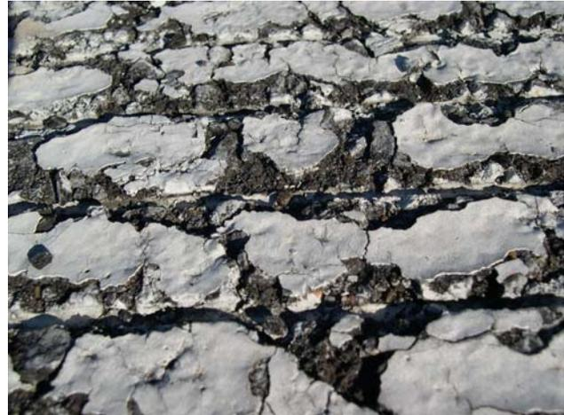
**FIGURE 5-23. EVIDENCE OF BOTH PAINT AND ASPHALT CRACKING INDICATES PRE-EXISTING CONDITION.**
