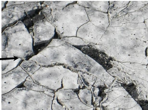
**FIGURE 6-9. THICK COATING CRACKED, CAUSING PAVEMENT TO CRACK AS WELL.**
