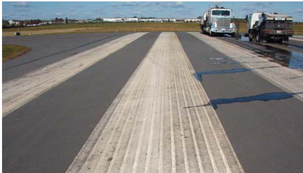
**FIGURE 4-1. BEFORE CLEANING LOOSE AND POORLY BONDED PAINT.**
