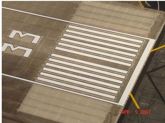
**FIGURE 5-33. THE VISIBLE SCAR IS CLEANED PAVEMENT.**
