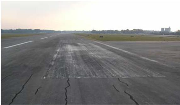
**FIGURE 4-16. BEFORE WATERBLASTING: ALGAE OBSCURE MARKING.**
