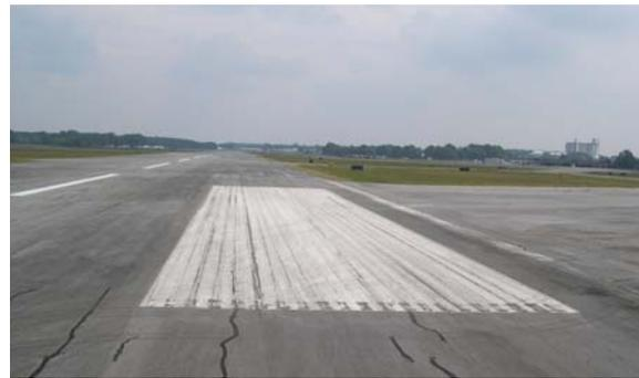
**FIGURE 4-17. AFTER WATERBLASTING, BUT BEFORE PAINTING.**
