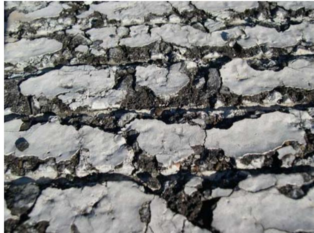
**FIGURE 4-5. MAGNIFIED PHOTO OF FIGURE 4-4 SHOWS CRACKED ASPHALT WHERE WATER INVADES.**
