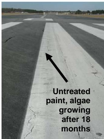
**FIGURE 4-18. PAINT USED WAS STANDARD TT-P-1952E.**
