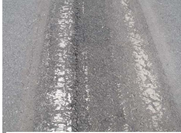
**FIGURE 5-30. REMOVAL OF MULTIPLE LAYERS ON DETERIORATED ASPHALT.**
