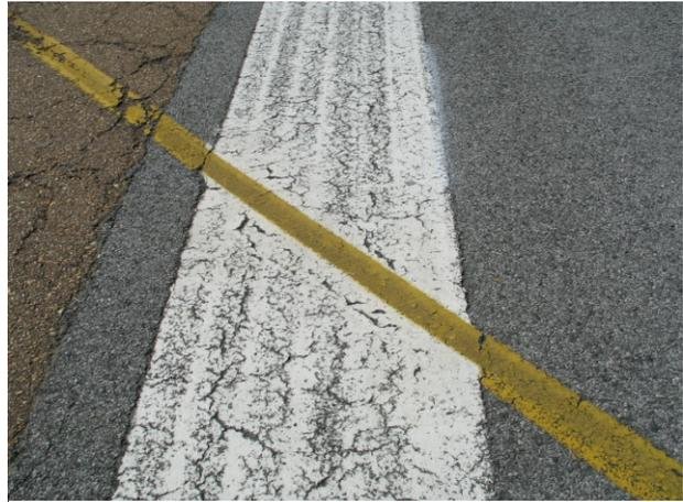
**FIGURE 5-3. CRACKED AND PEELING MARKINGS – REMOVE 85 PERCENT.**
