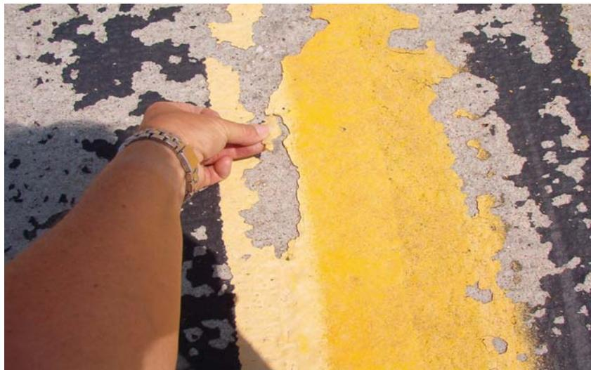
**FIGURE 4-42. LOOSE PAINT FOUND AFTER SURFACE PREPARATION. PAINT REMOVAL IS REQUIRED.**
